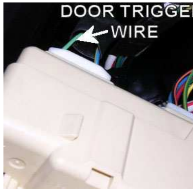
Pictured is the location of the door trigger wire behind the fuse box of a 2001 Toyota 4Runner.
