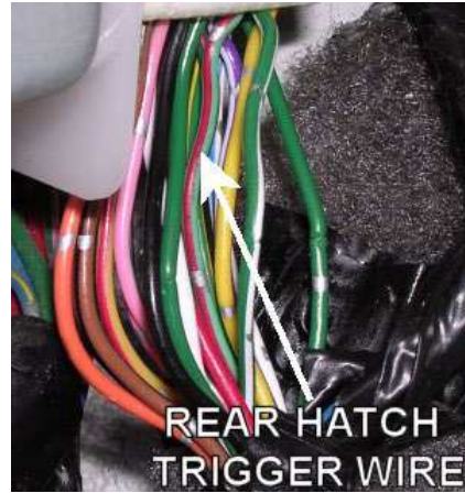
This picture shows the location of the rear hatch trigger wire in the driver's kick panel in a 2001 Toyota 4Runner.
